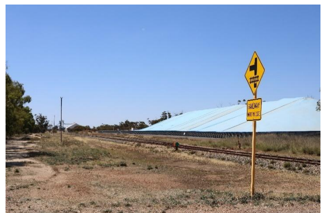
Figure 5-27 Grain siding at Muntadgin
