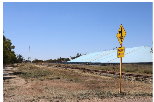
Figure 5-7 Railway and siding at Muntadgin
