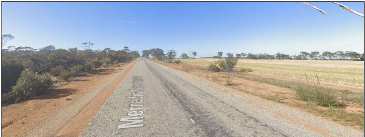
Figure 2-5 Merredin-Narembeen Road looking south (Google Street View, 2025)
