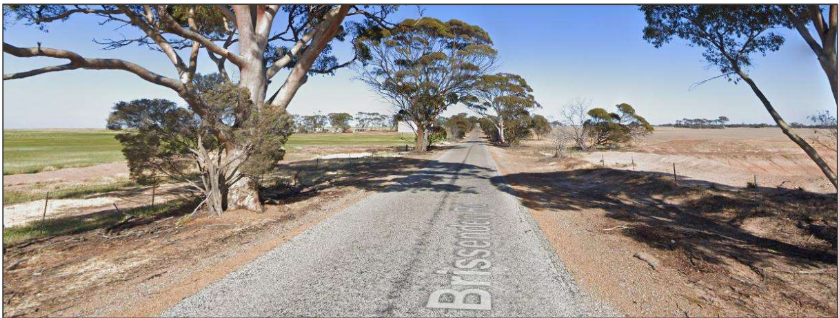
Figure 2-6 Brissenden Road looking west (Google Street View, 2025)
