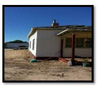
The walls on the west and east side are collapsing and daylight can be seen through the eaves and into the roof space from the front veranda.
