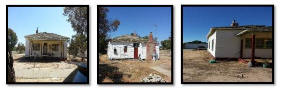
The walls on the west and east side are collapsing and daylight can be seen through the eaves and into the roof space from the front veranda.
