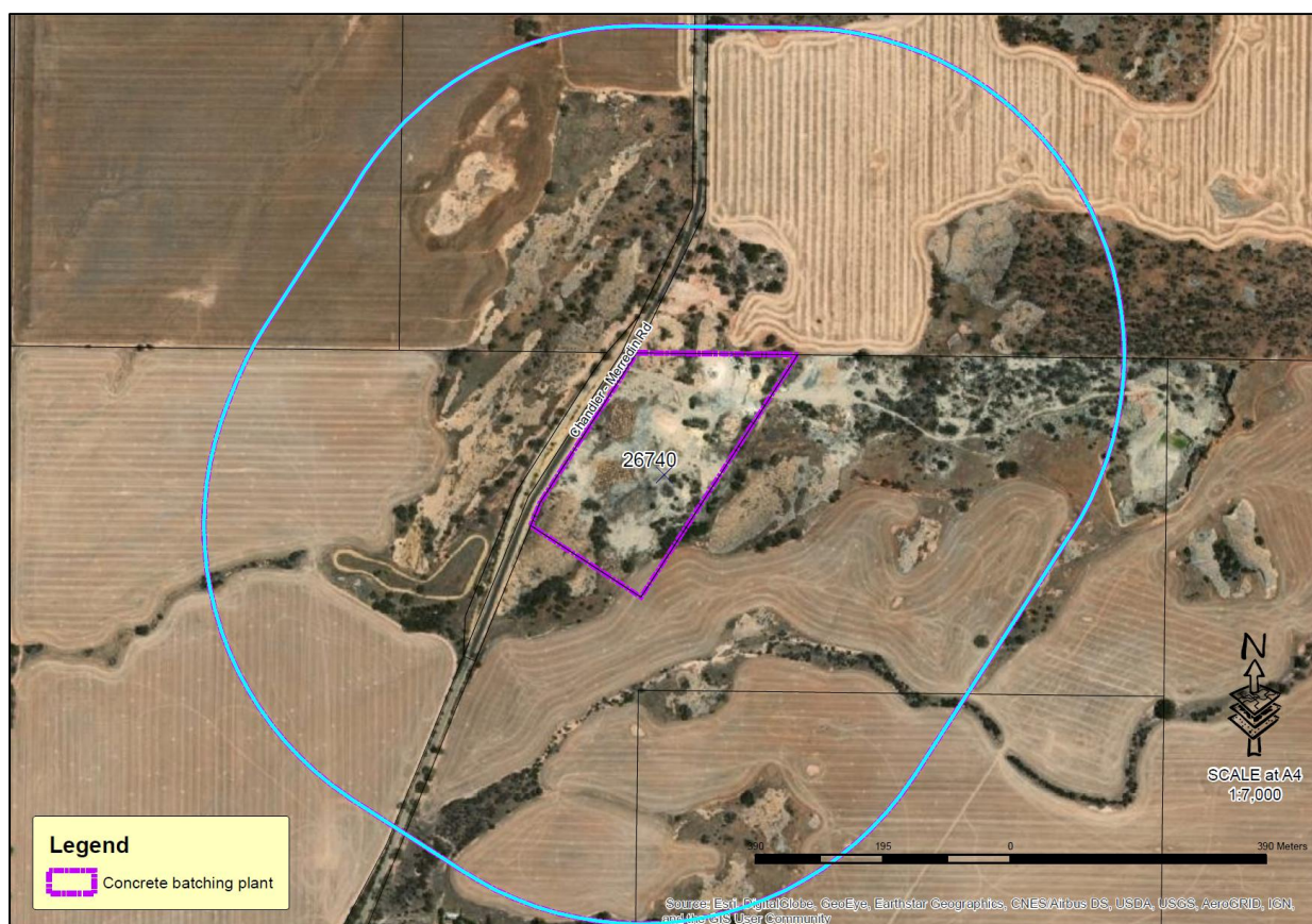
FIGURE 15 – CONCRETE BATCHING PLANT
