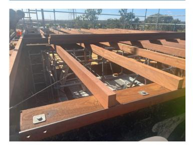
During a recent visit up the Water Tower, the timber work for the roof was in the final stages of completion, and the contractors were finalising the top bracing works.
