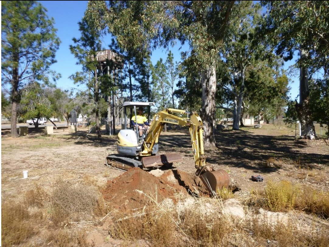
Photo 3. Test Location 01 (TP1), Sub-surface probing by using an excavator
