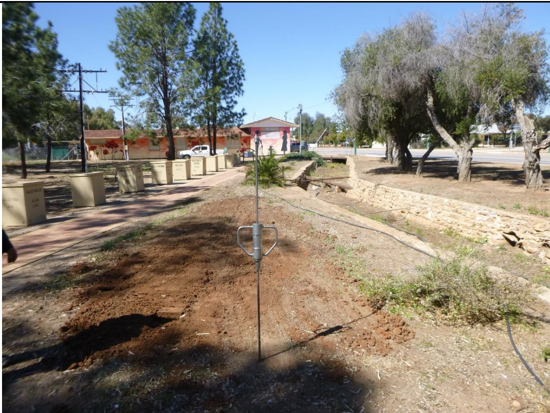
Photo 6. Test Location 01 (DCP1), Testing by Dynamic Cone Penetrometer
