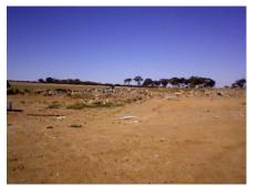
All inert materials will be sorted and removed from this area where a cell will be created. The view is north east towards the back of the hill. The overburden created can be used to cap cells and permit the creation of contours to drain water from the site.
