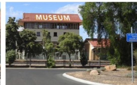
Example showing the inclusion of the painted sign onto the roof of the Signal Box.
