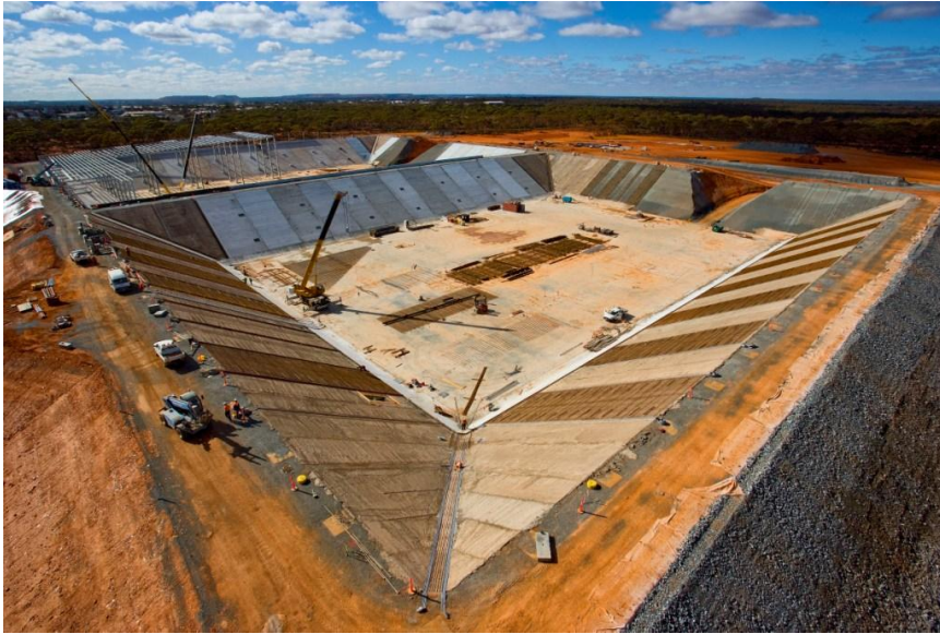
Existing Binduli Reservoir during construction
