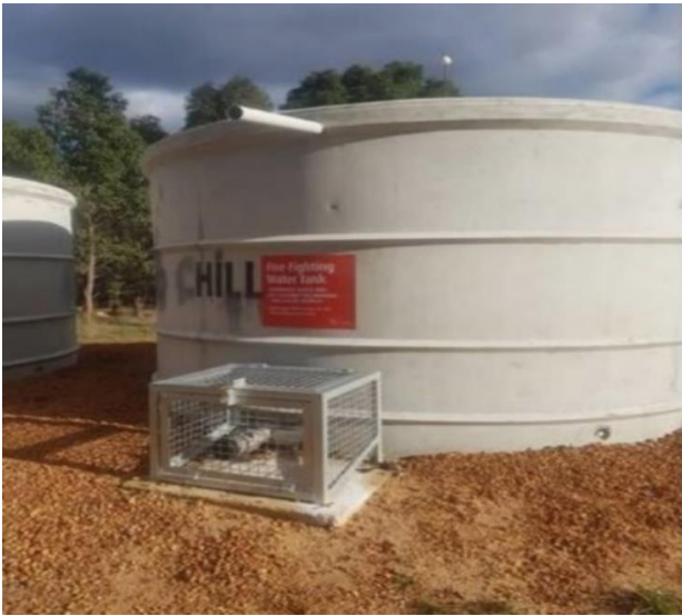
Strategic 47,000 Litre Concrete Tank & Protected Fittings
