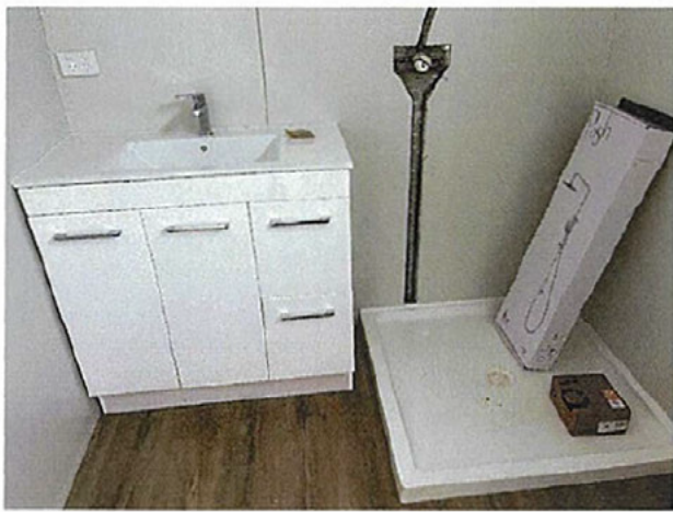
PHOTO OF BATHROOM FIT-OUT (STILL TO BE COMPLETED)
