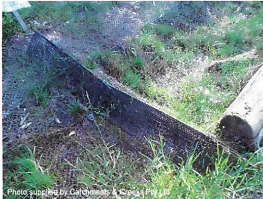
Photo 5 – Triangular ditch checks
