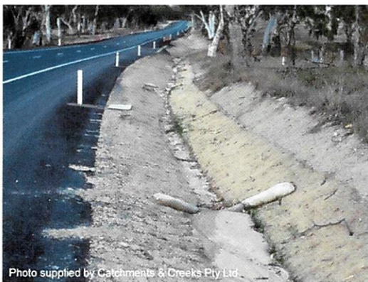
Photo 1 – Sandbag check dams
