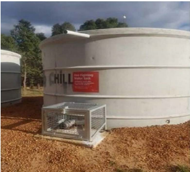
Strategic 47,000 Litre Concrete Tank & Protected Fittings
