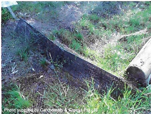
Photo 5 – Triangular ditch checks
