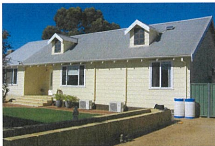
PHOTO OF THE EXISTING
