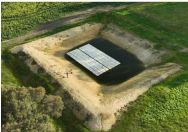
Figure 2: Left-Daisy Dam Cover at Kojonup exploring options for reducing evaporation. Right- Farm water planning with growers.
