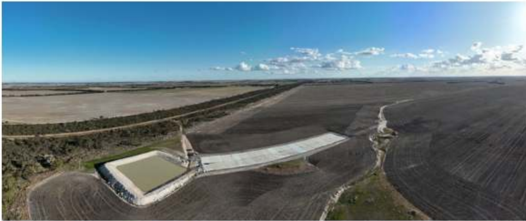
Figure 1: Recycled CBH Tarp Catchment at Jacup- increasing run-off into the dam.
